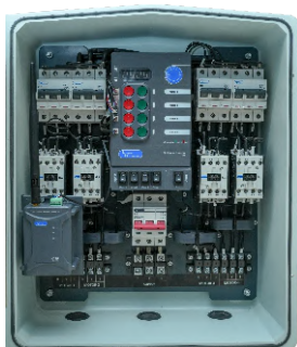
Interior View of xMU-GiA
