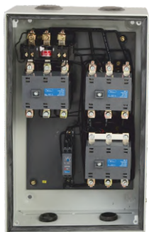
Interior View of ML FASD
