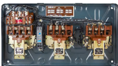
Interior View of MK2 FASD
